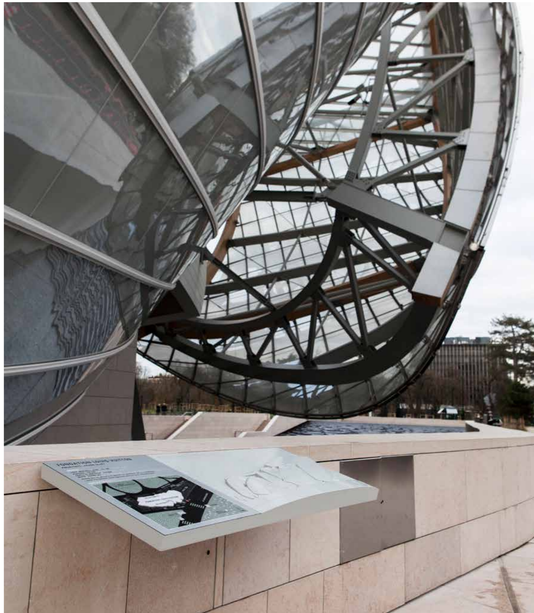
Louis Vuitton Foundation, France Tactile orientation solutions
